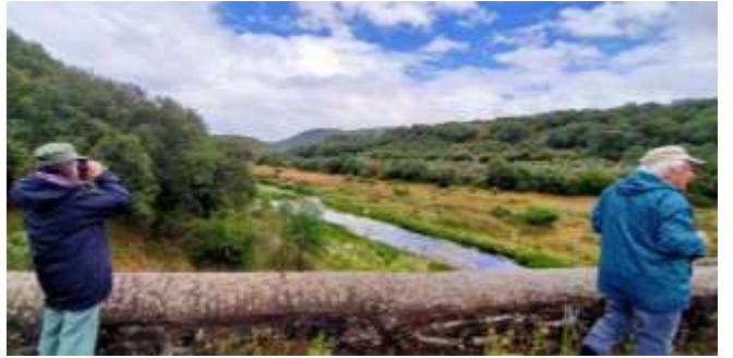
Bridge over the river Alagon
